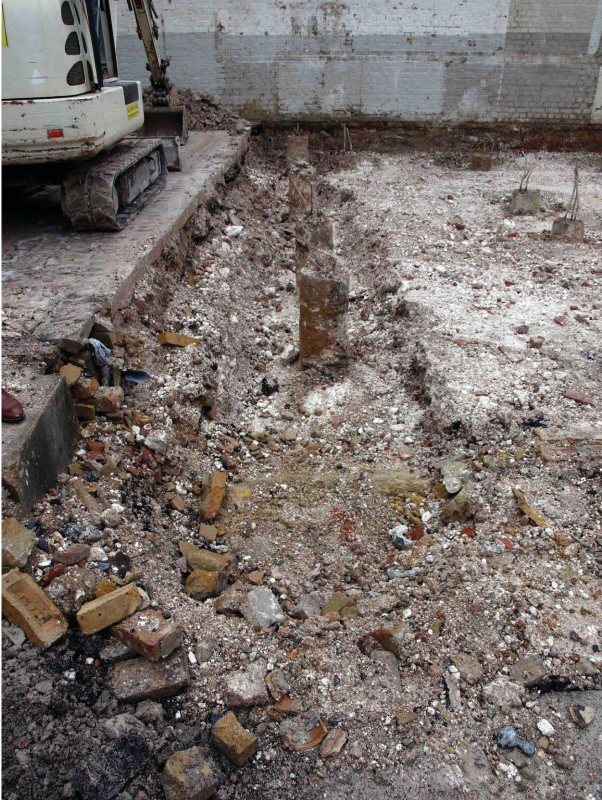
Plate 3. Removal of previous building slab and extent and depth of excavation
