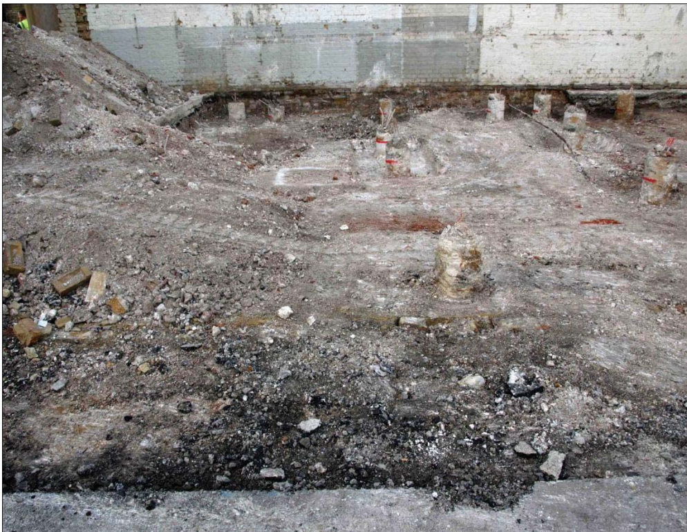
Plate 1. View of site
